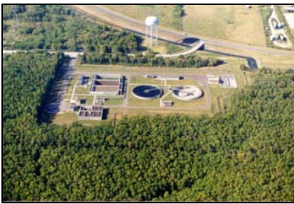
Arial Photograph of Groves WWTP
